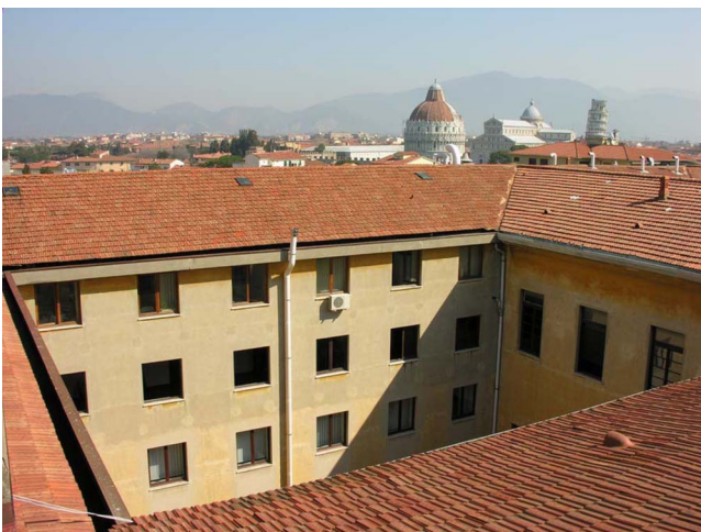
Fig. 2. Construction site with the background of the Cathedral Square and the Leaning Tower
